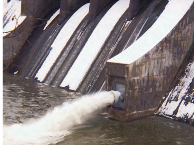
Berlin Lake Dam, Ohio, USA—Two Ring Jet Valves (36") and Eight Ball Valves (36").
