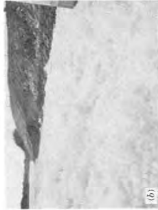
72-inch left valve discharging 100 percent open 1,750 cfs approx. - T. W. elev. 301.83 - T. W. elev. 182.7 Compare with Figures 26 & 27
