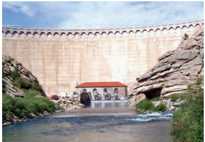
Eleven Mile Dam, Colorado, USA—View from downstream.
