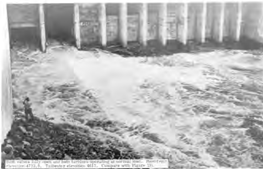
FIG. 22.—BOYSEN DAM OUTLET WORKS DISCHARGING 1344 CFS
