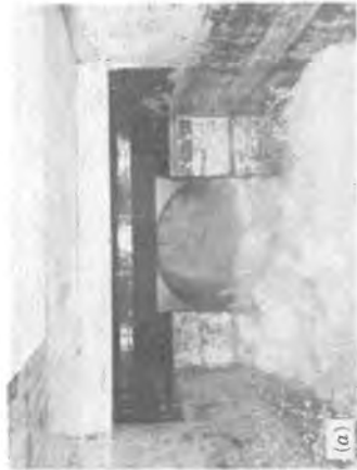
72-inch left valve discharging 100 percent open 1,750 cfs approx. - T. W. elev. 301.83 - T. W. elev. 182.7 Compare with Figures 26 & 27
