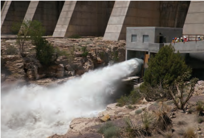
Pueblo Dam, Colorado, USA—One Ring Jet Valve (60") and One Rotovalve® Cone Valve (60").
