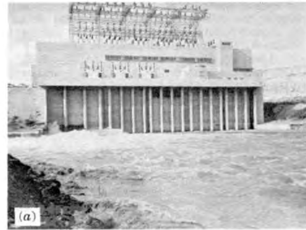
90-inch outlet works valves open 100 percent discharging 4,500 cfs approx. - T. W. elev. 183.6. Turbine gates 72 percent open - 100 percent load.
