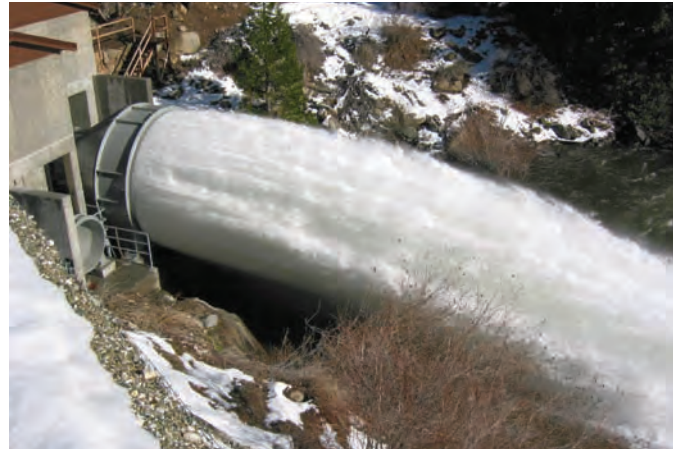
Salt River and Lower Bear Reservoirs, California, USA—Four Howell-Bunger Valves, with stationary hoods (18", 24", 60", 78").
